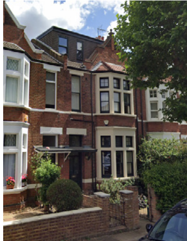
Figure 31: Dormer extension, Dundonald Road
