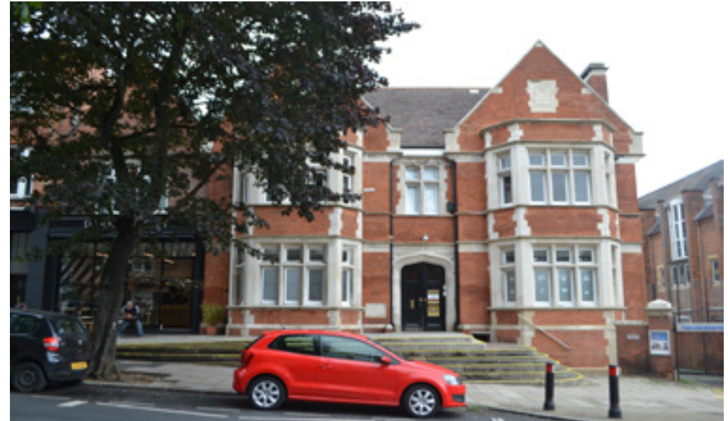
Figure 25: 131 Salusbury Road (old electricity dept.)
